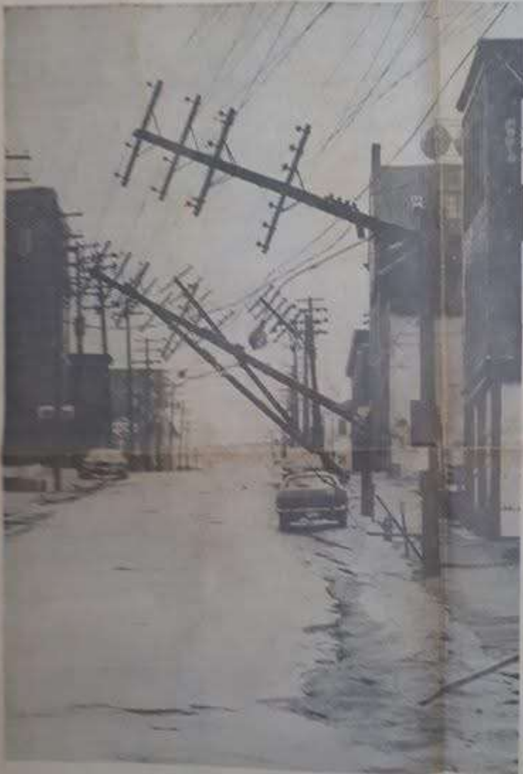
Street poles along uppermost Union Street snapped
