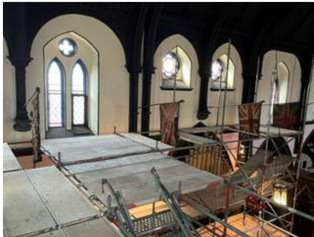
South Side of Sanctuary
